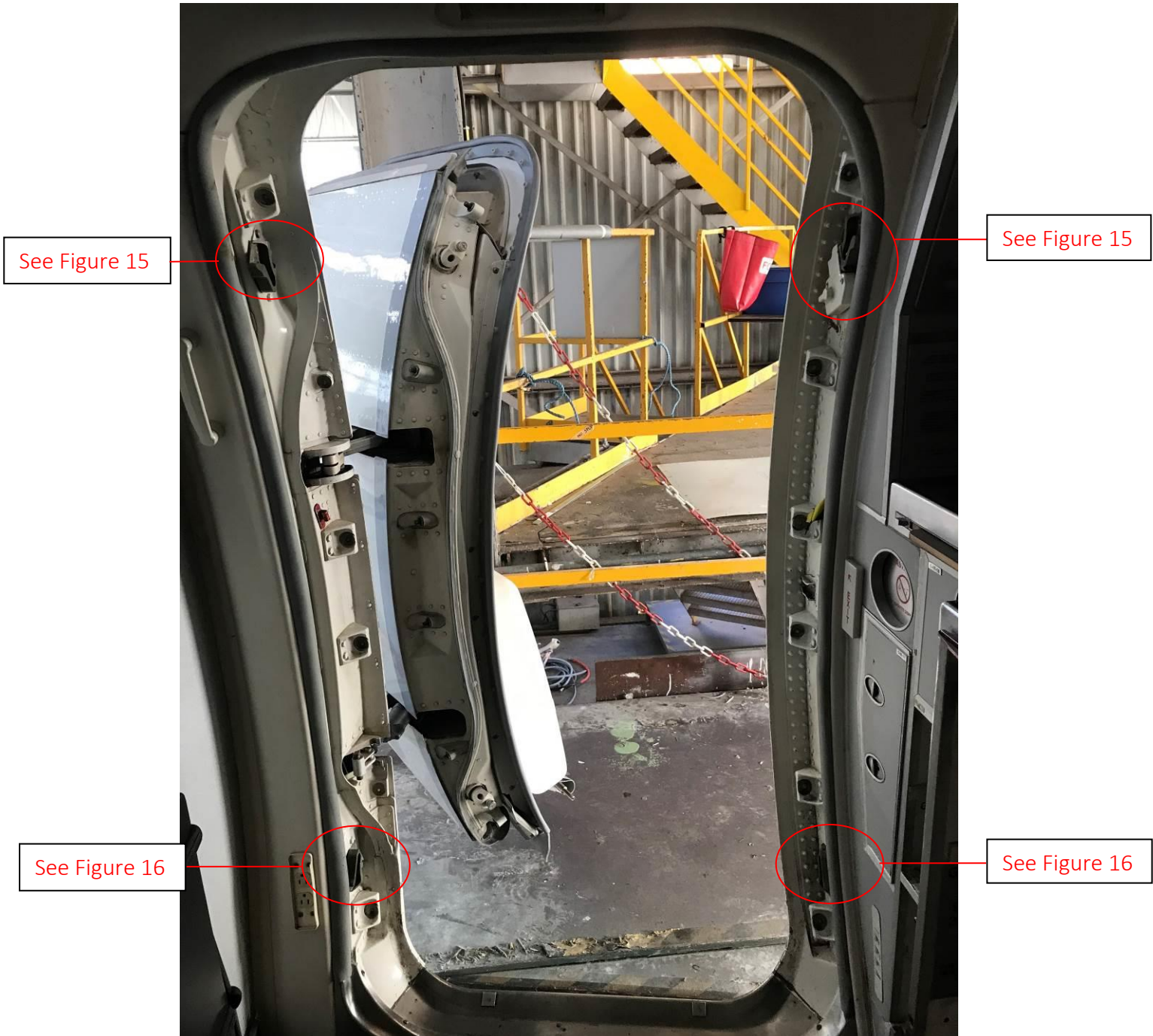
Figure 14 – Forward Service Door Bracket Positions. (Note: Brackets are the same for Aft Entry and Aft Service Door)
