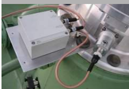
Bushing adapter and coupling unit
