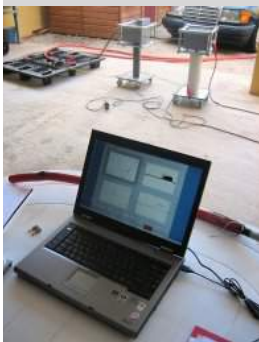
On-site cable testing
